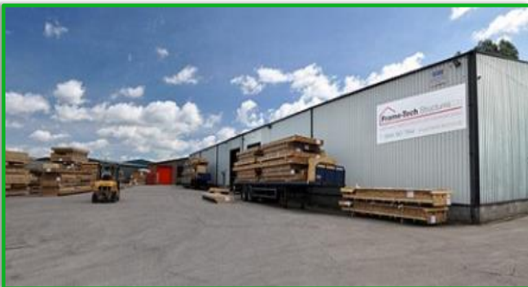
Frame-Tech Structures Ltd Lock Way, Ravensthorpe, Dewsbury WF13 3SX, United Kingdom
